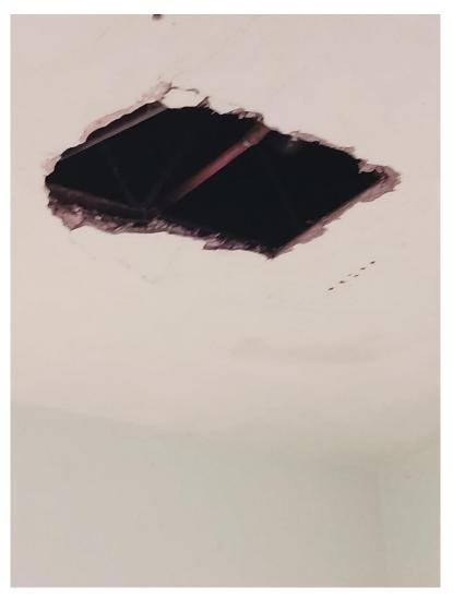
We patched the hole and repainted the ceiling in that area to match existing pain. Following pictures show Sir Knight Kevin Patrick at work and the patch prior to taping, mudding and painting.
